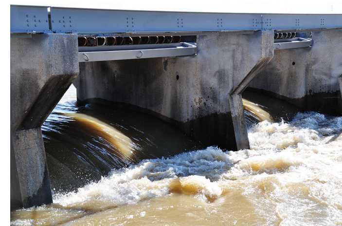
The Bonnet Carré Spillway, just upstream of New Orleans, diverts floodwater from the Mississippi River and protects the city. It has been opened 6 times in the last decade. Gulf Restoration Network/HealthyGulf.org.
