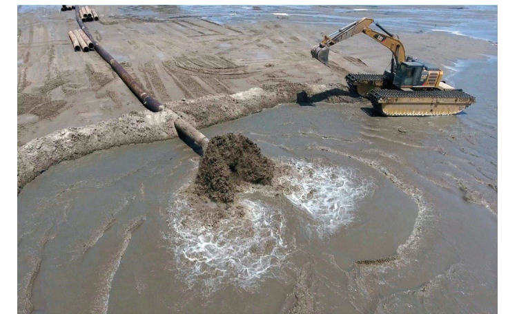
Dredge materials have been used to help rebuild coastal Louisiana. P.J. Hahn, Pelican Coast Consulting and the Big River Coalition.
